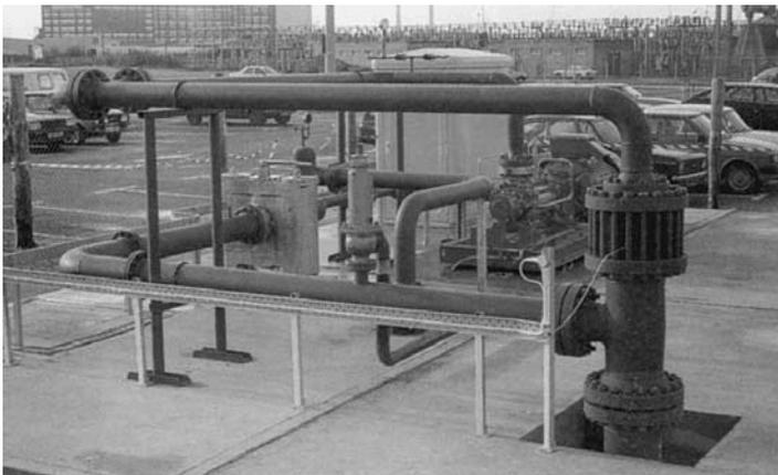
4.33 Southampton geothermal well head, brine pump and filter (reproduced by courtesy of Southampton Geothermal Heating Company).
