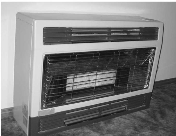
4.1 Gas radiant and fan convector room heater.
