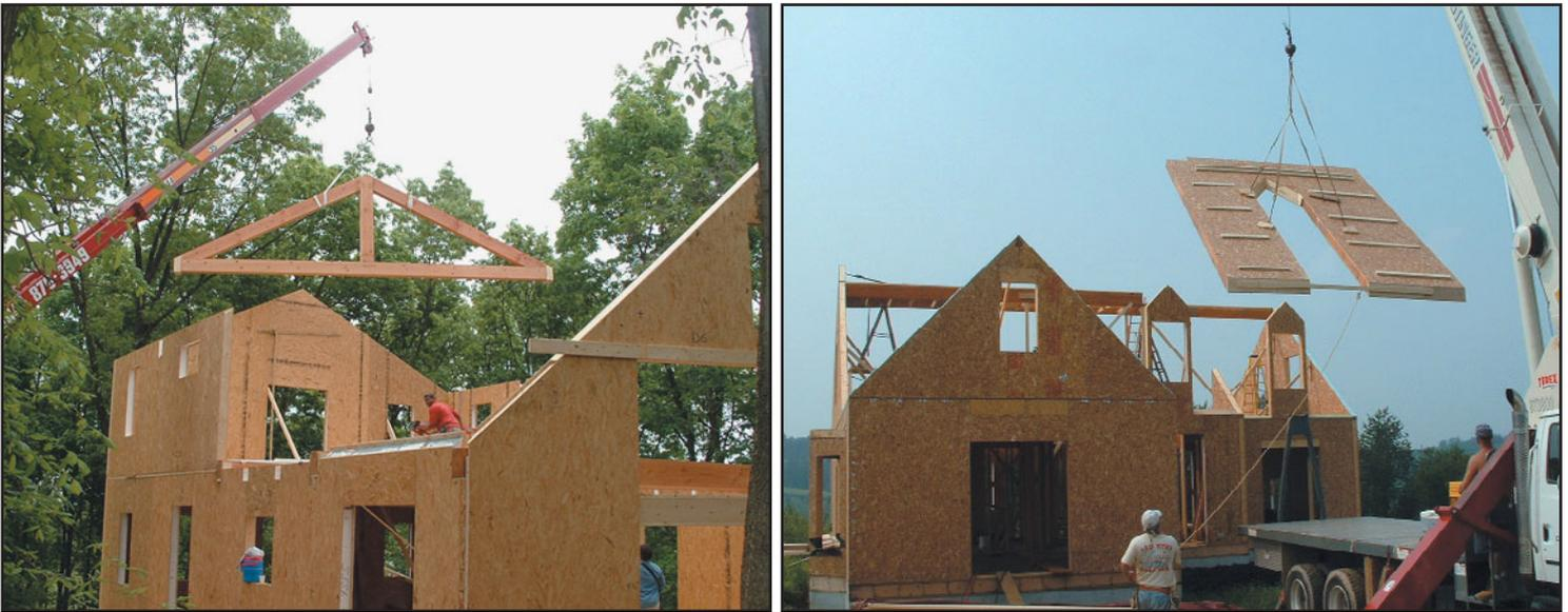
**FIGURE 17.1** Two examples of typical structural insulated panel buildings under construction. (Photos courtesy of the Structural Insulated Panel Association [SIPA])
